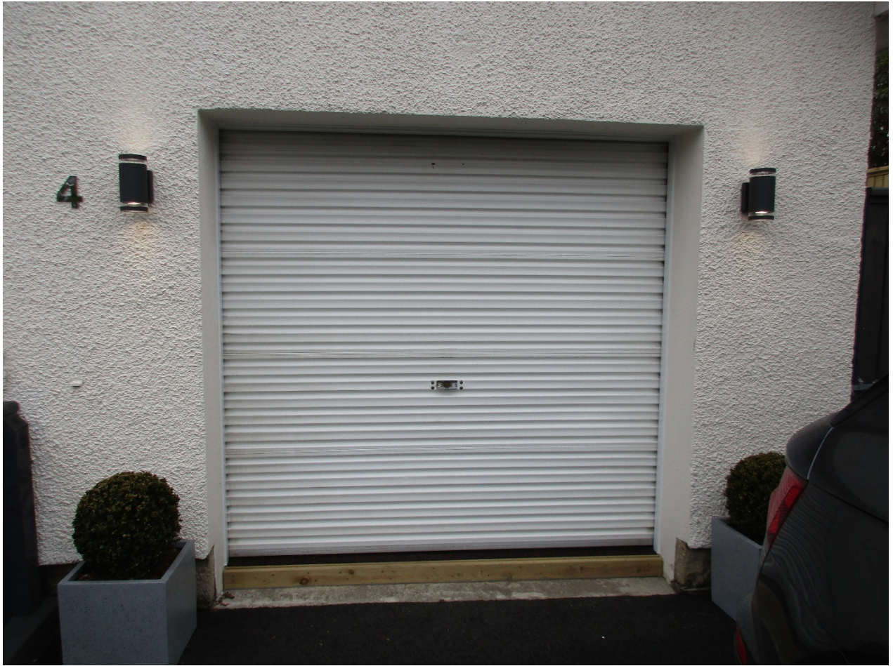
GARAGE FRONTAGE SHOWING ROLLER SHUTTERS CLOSED
